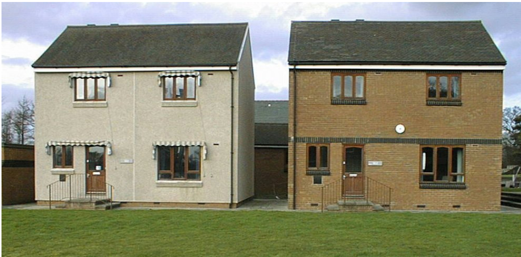
Figure 1 Front view of the 'Standard' BRE Test Houses. Reference House 1 on the left and Test House 2 on the right
